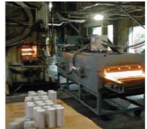
Electric IR System to Pre-Heat Aluminum Billets
