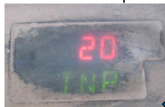
Damper Controlled at 20% Open
