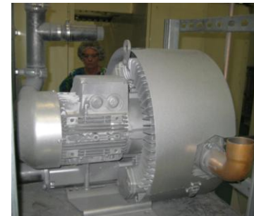
Local Blower on Process Line
