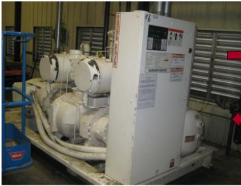
300 HP Gardner Denver Air Compressor
