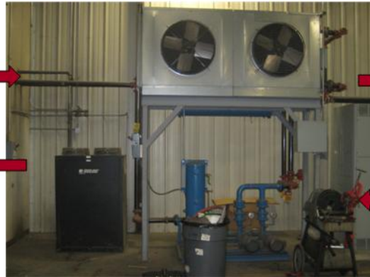
Heat Reclamation in Winter (110°F Air) (installed cost ~ $25k)
